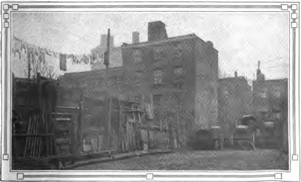
A back view of Trinity tenements. An owner has here torn down his house rather than let it fall into Trinity's possession when the lease expired
