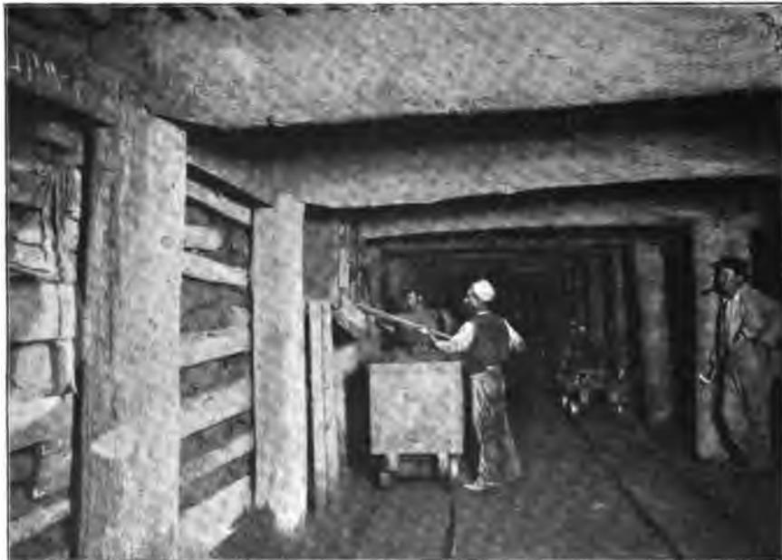
FIG. 38.—SOUTH DRIVE NO. 2 LEVEL, NO. 4 LODE (SHOWING TIMBERING), GOLDEN HORSE-SHOE.
