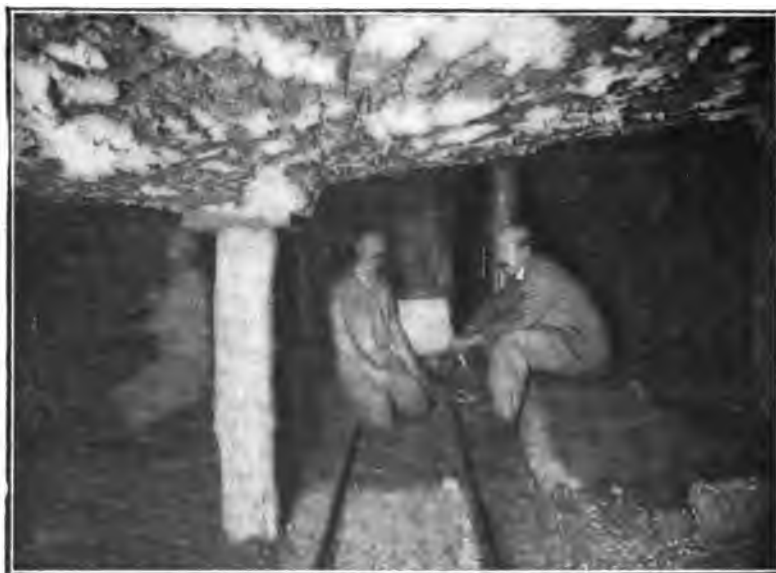
FIG. 21.—UNDERGROUND WORKING IN AN ALLUVIAL CLAIM.
