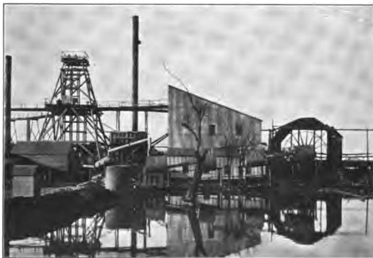
FIG. 49.—THE GOLDEN HORSE-SHOE WORKS (SHOWING TAILINGS-WHEEL).
