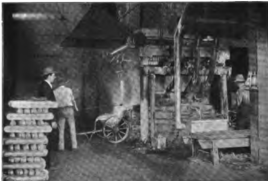
FIG. 65.—WATER JACKET FURNACE, GOLDEN HORSE-SHOE WORKS.
