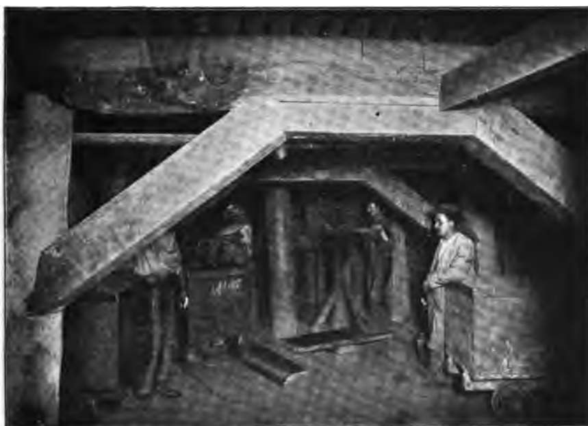
FIG. 39.—JUNCTION OF CROSS-CUT AND NO. 3 LODGE NO 1 LEVEL, GOLDEN HORSE-SHOE.
