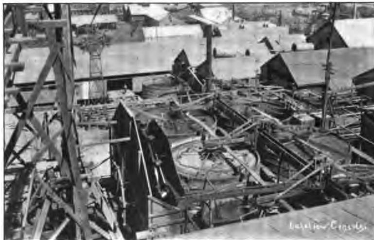
FIG. 52.—THE LAKE VIEW CONSOLS CYANIDE PLANT (SHOWING VATS WITH BUTTERS AND MEIN'S DISTRIBUTORS).
