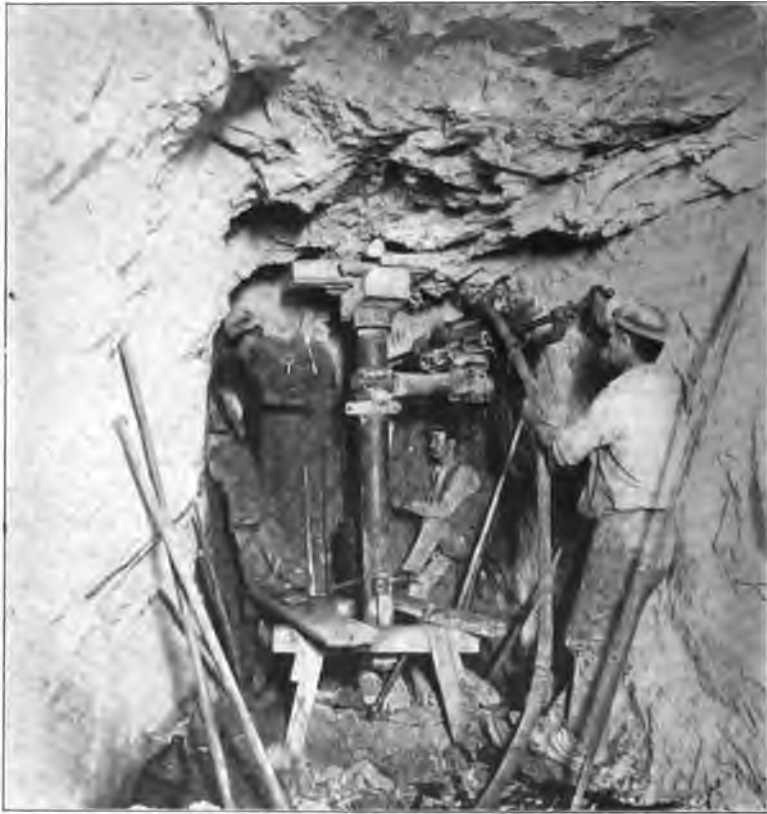
FIG. 31.—MACHINE DRILLS AT FACE, 200-FOOT LEVEL, LAKE VIEW CONSOLS.
