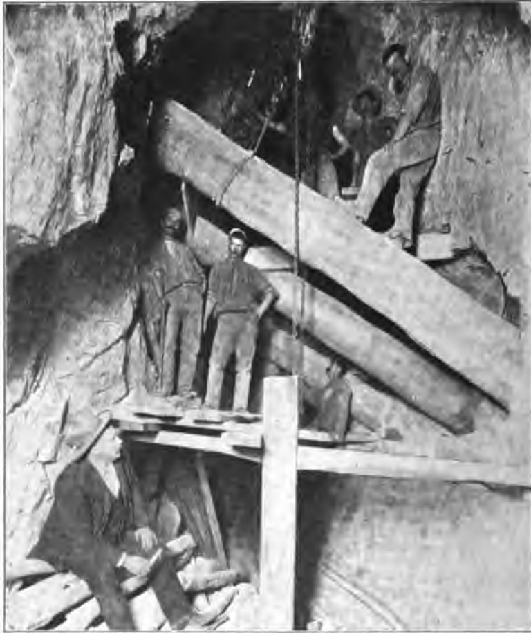
FIG. 36.—“STULL”-TIMBERING, LAKE VIEW CONSOLS.
