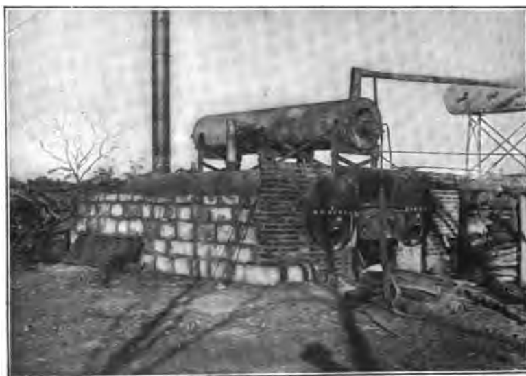
FIG. 25.—CONDENSER AT THE IRON KING MINE, KALGOOLIE. (By courtesy of T. A. Rickard.)
