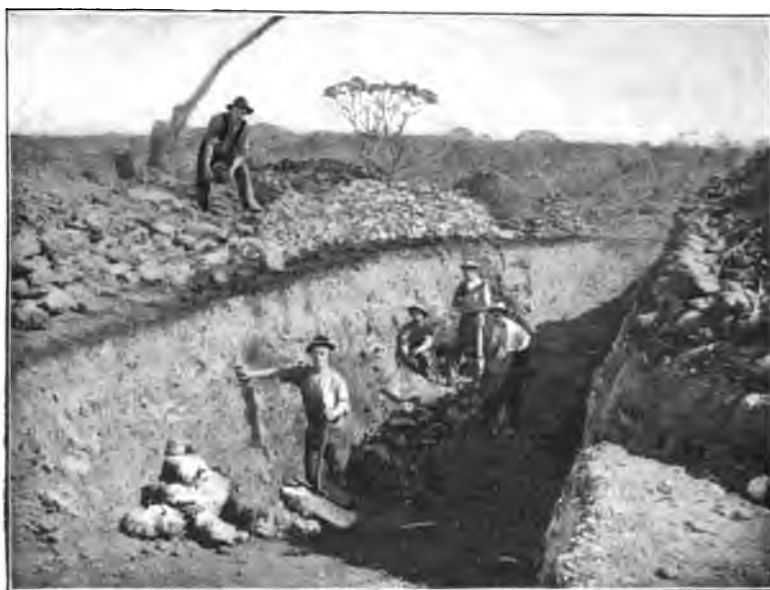
FIG. 19.—AN "OPEN-CUT" AT KANOWNA. (Reproduced by courtesy of The Financial Times .)
