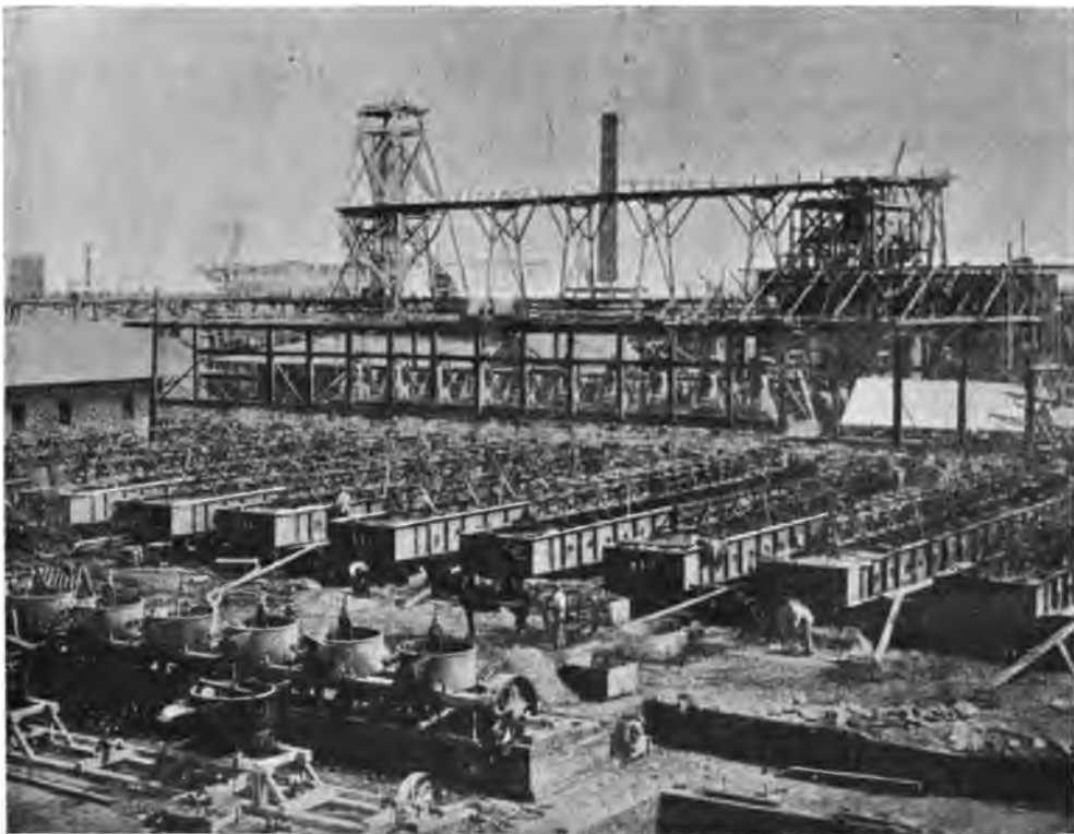
FIG. 59.—THE SULPHIDE PLANT IN COURSE OF ERECTION, EDWARDS' FURNACES AND PANS.
