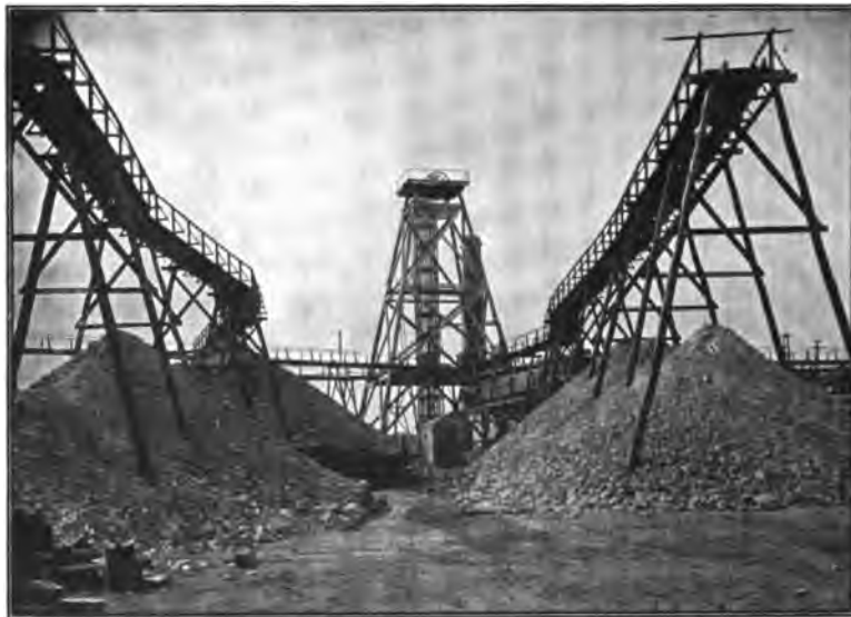
FIG. 29.—HEAD-GEAR, AND DUMPS, AT THE GREAT BOULDER MAIN SHAFT.
