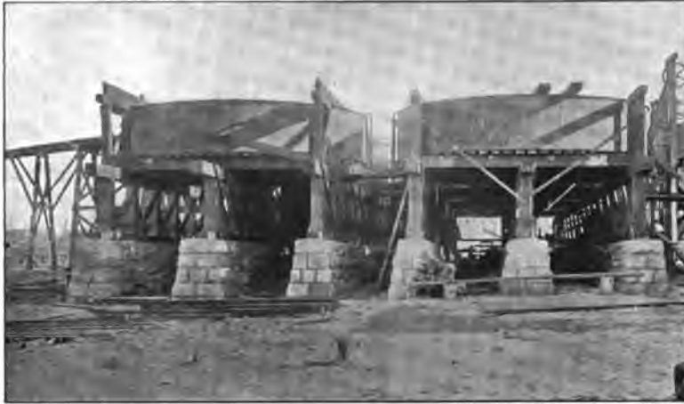
FIG. 51.—THE NORTH BOULDER CYANIDE VATS.
