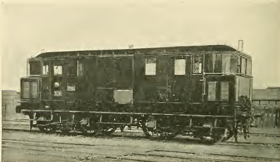
Fig. 281. "BAGGAGE CAR" TYPE OF PARIS-ORLEANS ELECTRIC LOCOMOTIVE.
