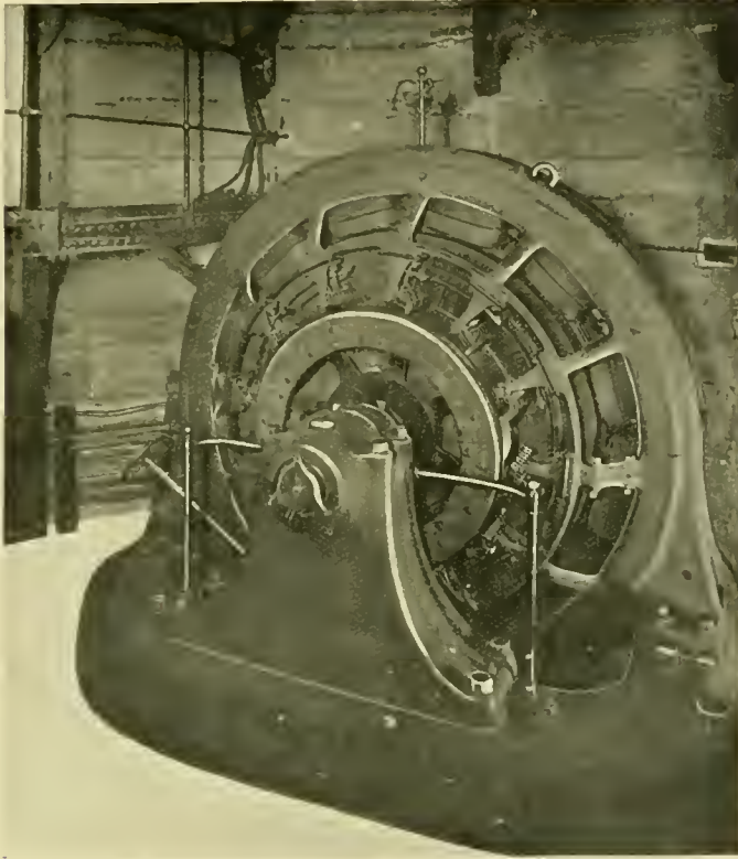
Fig. 190. CENTRAL LONDON RAILWAY: 900-K.W. ROTARY CONVERTER.
