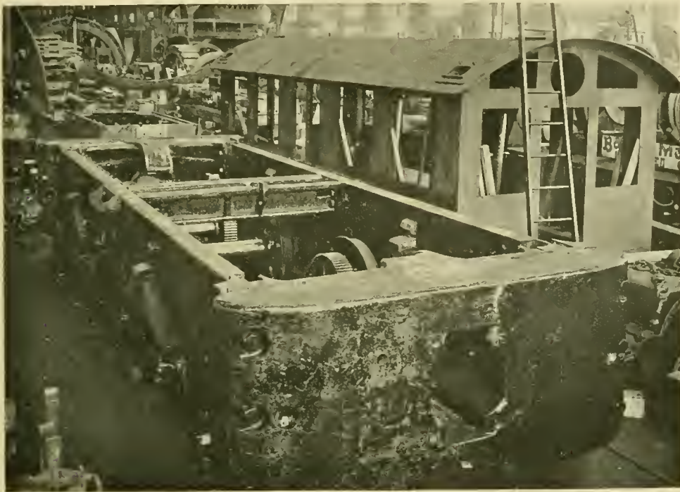
Fig. 272. FRAME OF ONE-UNIT OF BALTIMORE AND OHIO 1903 ELECTRIC LOCOMOTIVE.
