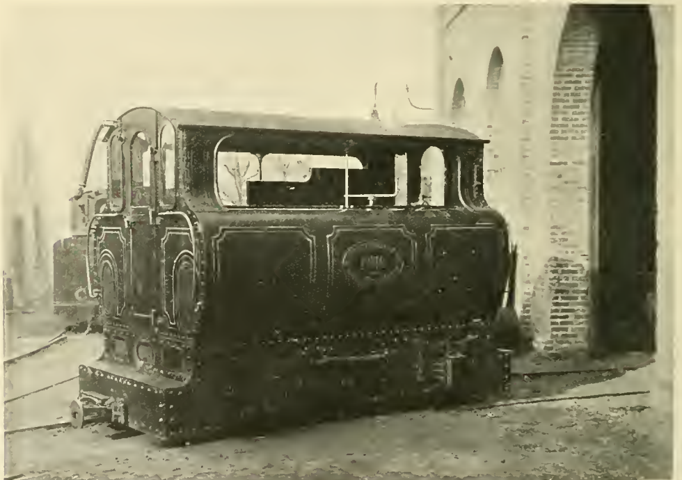
Fig. 275. CITY AND SOUTH LONDON GEARLESS LOCOMOTIVE.
