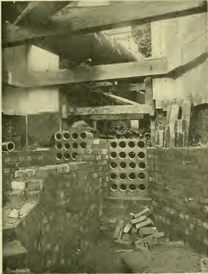
Fig. 142. DISTRICT RAILWAY: MANHOLE IN TRANSMISSION LINE UNDER CONSTRUCTION.
