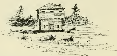
LOG WORK ON PORTAGE ROAD, 1764
